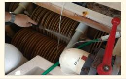
The Pool Pump Repairs are finally complete. New filters, vacuum gauge, a plunger valve and various leaks fixed. The aged equipment and COVID related supply chain problems prevented a timely repair. As well the original plunger valve cracked during repair and a new one caused a cost overrun. However, the pool pump equipment is again back to leak free operations.
